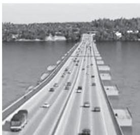
Pontoons jut out from bridge
